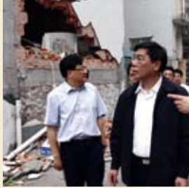
姜建清董事长查看本行绵竹分行受损情况 Chairman Jiang Jianqing is inspecting the damage of Mianzhu Branch
