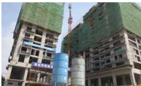
本行陕西分行支持的保障房建设项目 The affordable housing project supported by Shaanxi Branch
