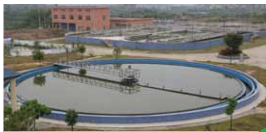
本行广东分行营业部提供融资支持的污水处理项目 Guangdong Branch Banking Department provided financing to sewage treatment project
