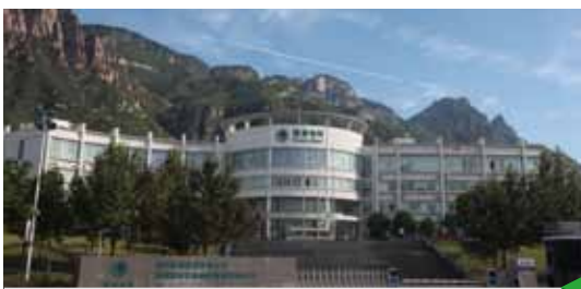
本行河南分行支持某抽水蓄能电站项目建设 A pump storage power station project supported by Henan Branch
