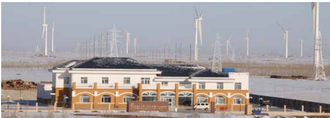
本行内蒙古分行支持的风电项目 The wind power plant project supported by Inner Mongolia Branch
