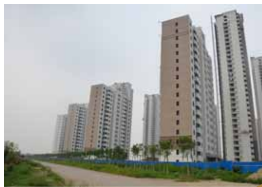
本行天津分行支持的安置用房项目 Resettlement housing project supported by Tianjin Branch
