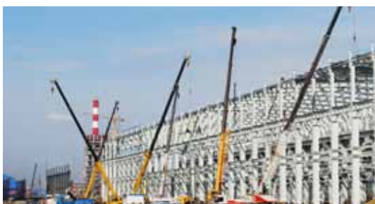
天津和谐型大功率机车检修基地项目现场 Project site of Tianjin Harmony High Power Locomotive Repair Base
