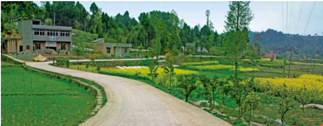
本行为通江县周子坪村铺就的致富路 A road leading Zhouziping Village of Tongjiang County to prosperity paved by the Bank
